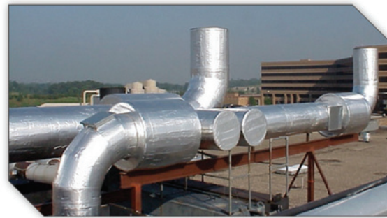
Mechanical insulation with laminate protective covering.
