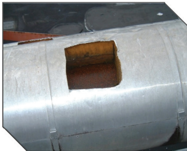
Example of cutting into an insulation system to inspect for corrosion under insulation
