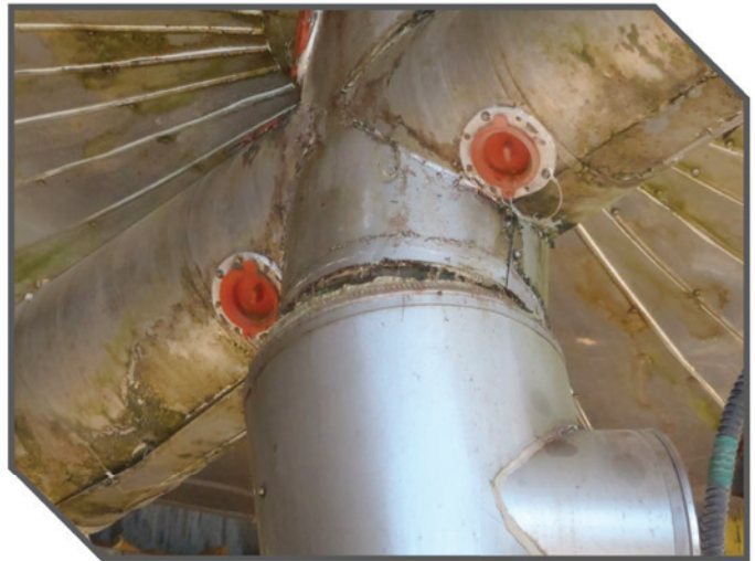
Example of using non-destructive inspector ports too late: Moisture had gotten into the system creating a host of problems—from mold development and separation of the insulation joints due to increased weight among other issues.
