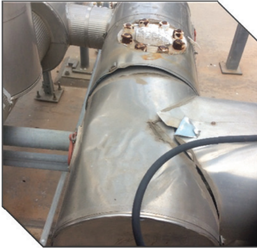
Example of mechanical abuse (probably foot traffic) damaging the insulation system opening joints for moisture intrusion
