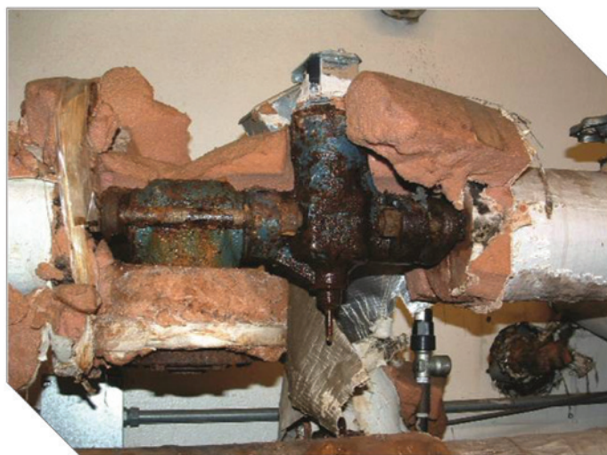
Corrosion under insulation
