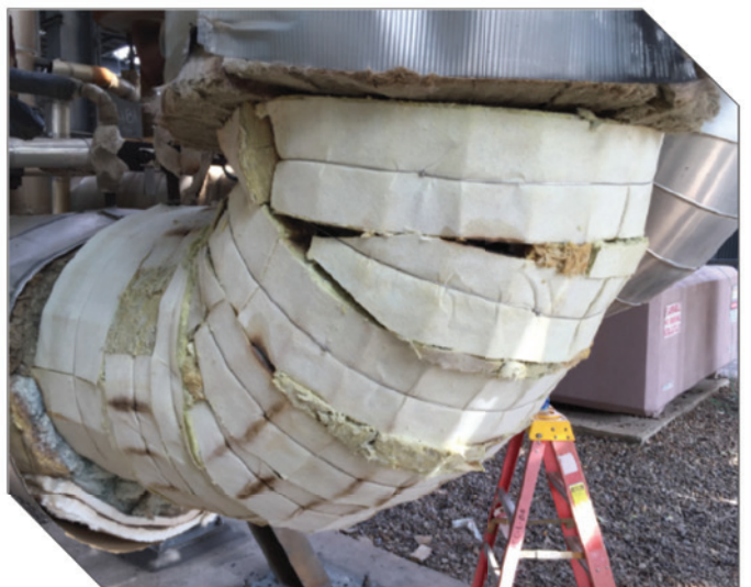
Example of unacceptable workmanship while trying to insulate an elbow
