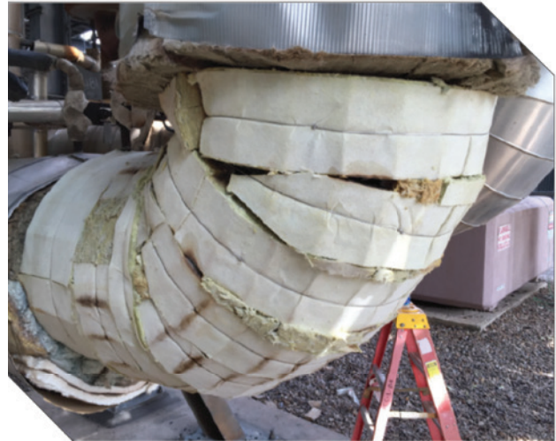
Example of improper insulation joints and installation of joint sealer
