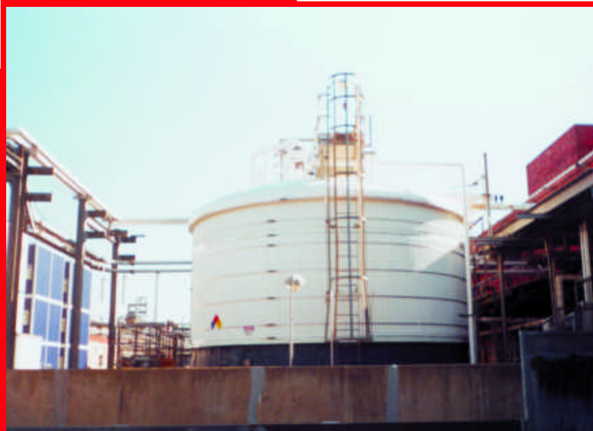
23.6 diameter x 16' high with dome roof. PVC corrugated panels and PVC tank heads. Photo courtesy of Proto Corp.
