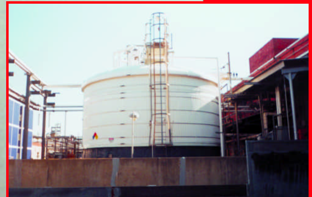
Corrugated panels and tank head. Photo courtesy of Proto Corp.
