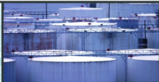
Associated specializes in the installation and maintenance of tank insulation panels.
