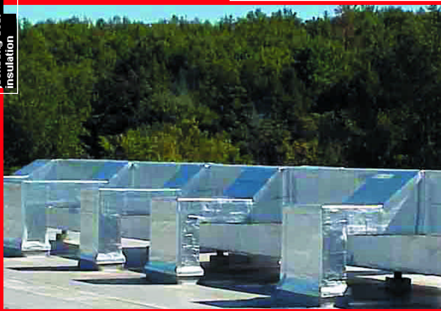
Aluminum jacketing over 2" FSK fiberglass board. Photo courtesy of Polyguard Products.
