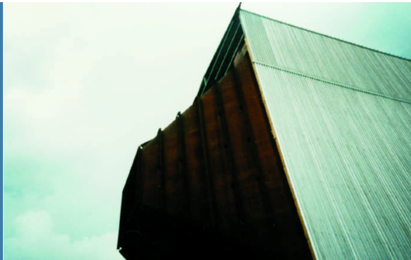
Partially insulated and lagged precipitator with the gas inlet nozzle unfinished.
