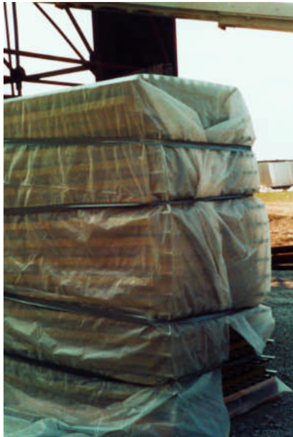
Pre-insulated lagging panels that are properly stored and weather protected, ready for installation.
