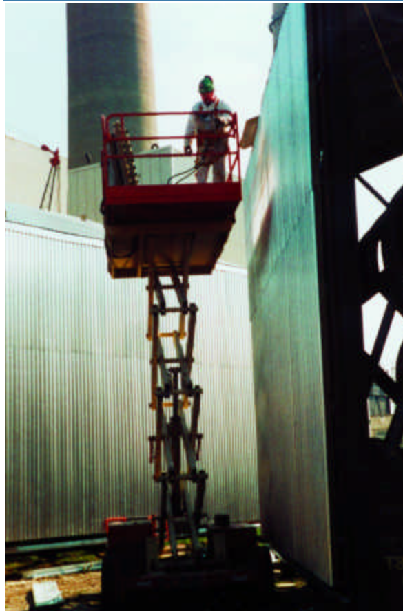
Field installation of pre-insulated lagging panels require special material handling requirements.
