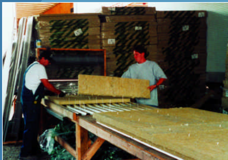
Field fabrication of pre-insulated lagging panels.
