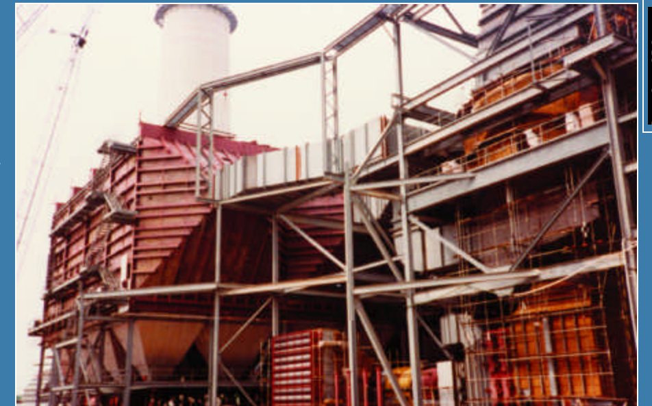
Precipitator and flues before insulation and lagging is installed
