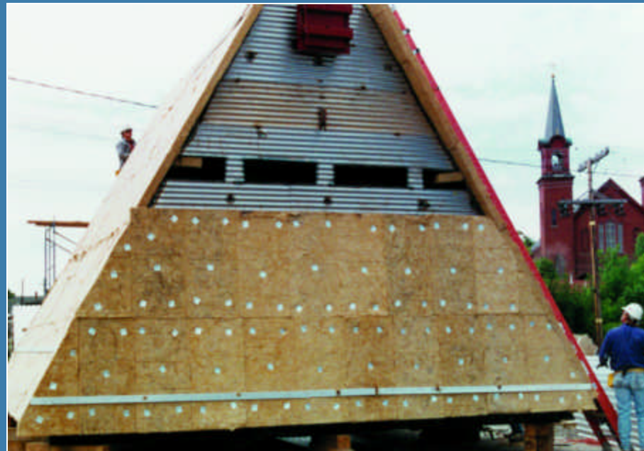
Ground installation of insulation and lagging on a precipitator hopper.
