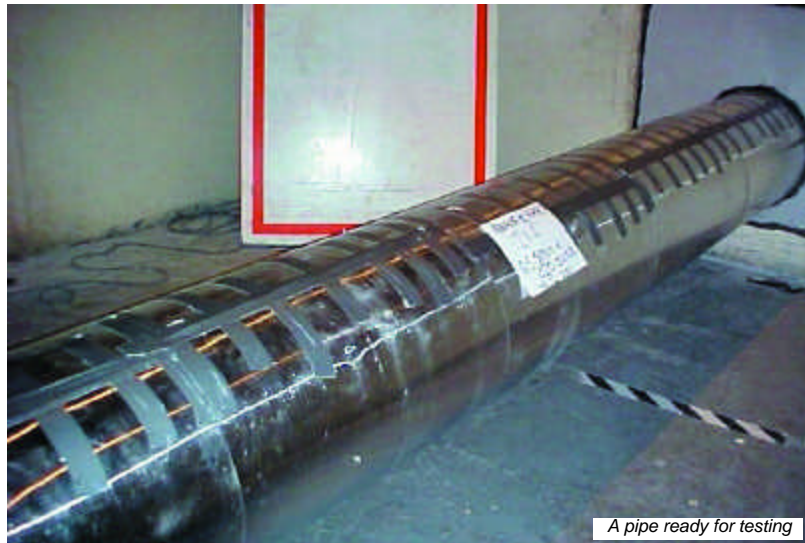
A pipe ready for testing
