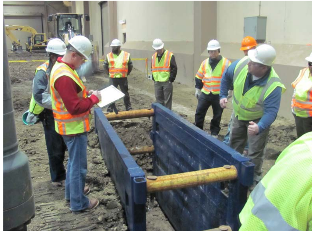
OTI #3010 – Excavation, Trenching & Soil Mechanics Course
